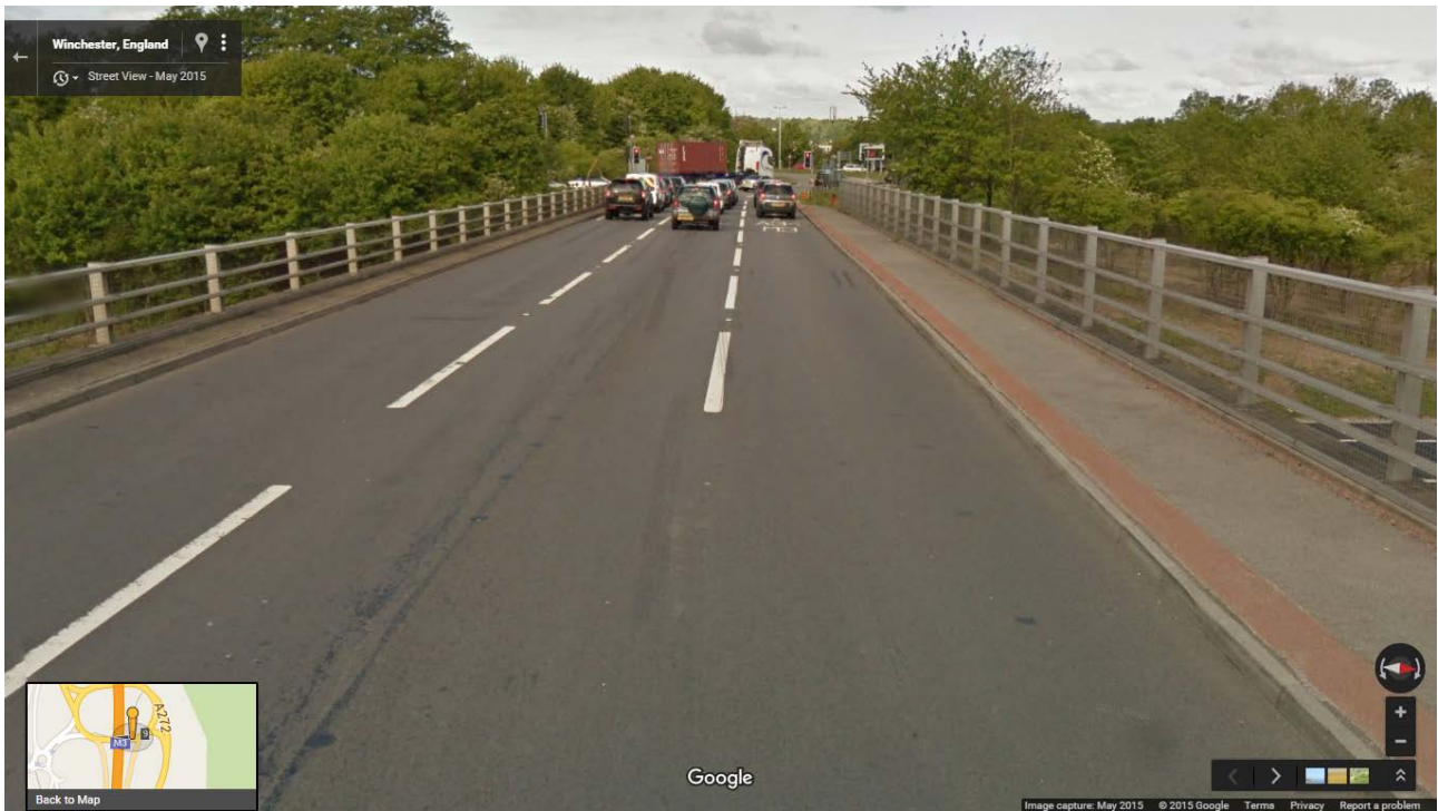
Above: Southern bridge lane markings realigned to three lanes © Google 2015
