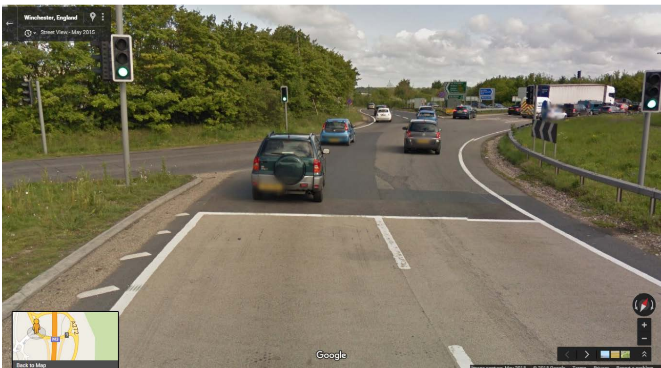
Above: Signals/stop line on the circulatory carriageway, junction with Easton Lane © Google 2015
